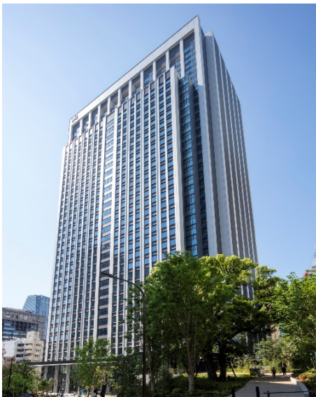
Kamiyacho Trust Tower ©Mori Trust Co., Ltd.
